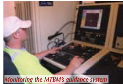
Monitoring the MTBM's guidance system
