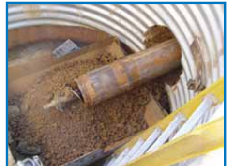
Spoils Discharged In Reception Shaft
