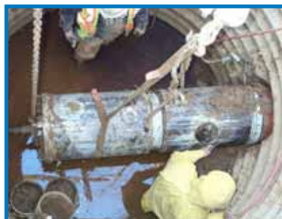
Drive Complete With Powered Cutter Head In Reception Shaft
