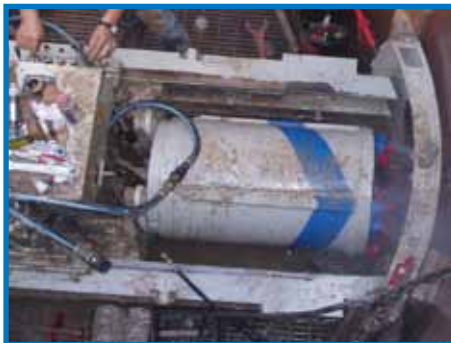
Powered Cutter Head In Launch Position
