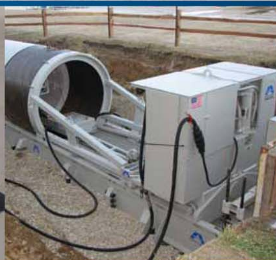
This photo shows how the yoke provides a 360-degree surface against the pipe to minimize point pressure and transfer thrust to the pipe.
