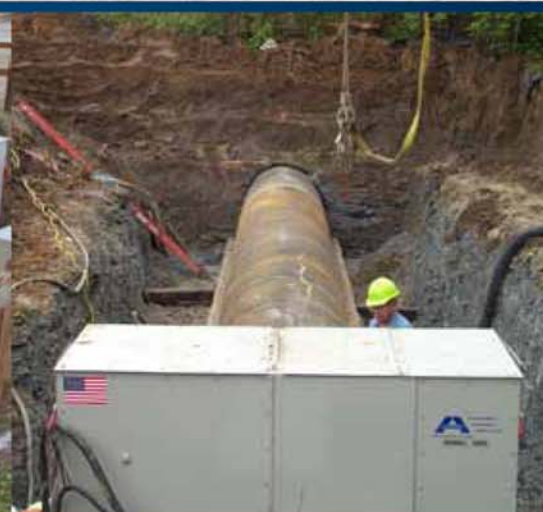
Extended skid base sections are available for long sections of pipe. Skids lengths range from 30-270 inches (762-6,858 mm).
