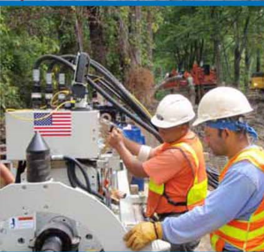
Operators of the 240A jacking frame have independent control of pipe jacking and rotation for smooth and continuous advancement.
