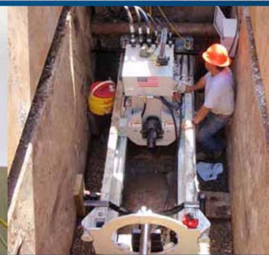
The 240A frame, when operated as a stand alone unit, can be used to expertly install up to 24-inch (610 mm) OD pipe.
