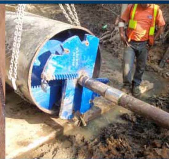
The Akkerman needle swivel is used in place of a weld-on reaming head to reduce thrust at the face of the bore.
