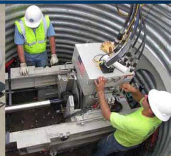
The 308A latching frame fits in a compact, 8-foot (2.4m) shaft.
