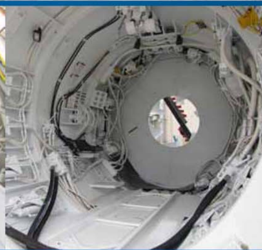
The interior of the TBM allows the operator full control over the forward movement and spoil removal processes while maintaining the cutter face excavation. The conveyor is installed in the center of the machine.
