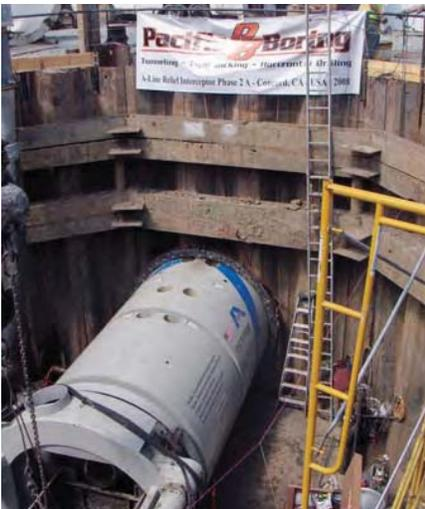
The 116-in. Akkerman EPBM will make way for 20-ft long sections of 96 ID tunnel pipe.
