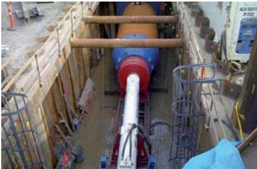
The HPD unit delivers 75,000-100,000kN of jacking pressure per blow
