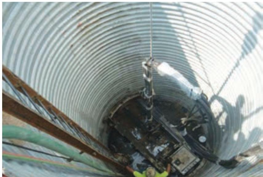
*Akkerman 308 guided boring machine set up in 9ft-diameter corrugated metal pipe*
