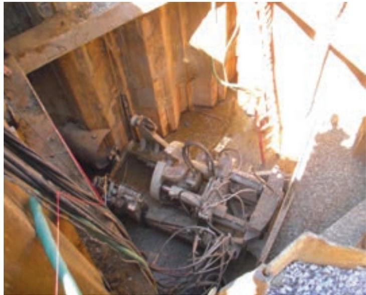
*Akkerman 4812 set-up in sheeted cell with casing and backstop in place*
