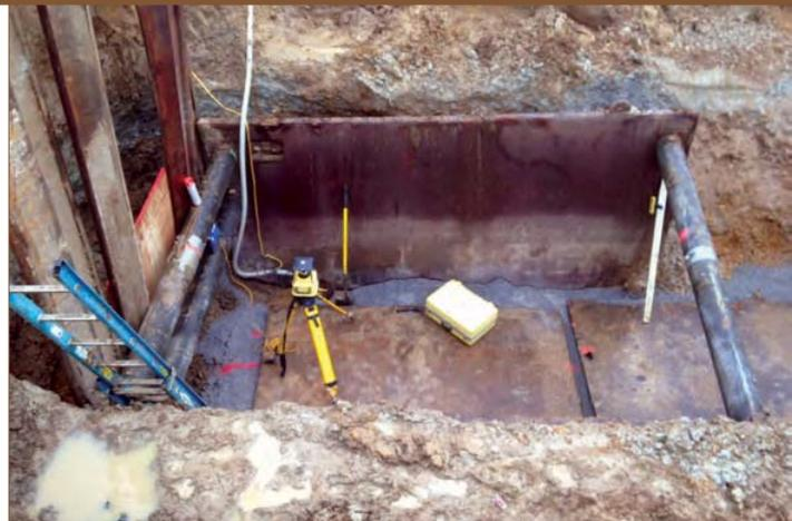
**ABOVE:** API CREW MEMBERS ARE SURVEYING THE SHAFT FLOOR PRIOR TO SETTING UP THE EQUIPMENT TO ENSURE THAT THE ELEVATION IS CORRECT.
