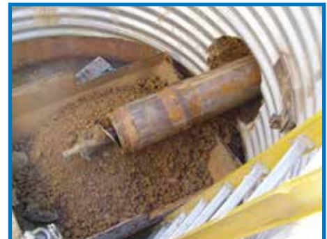
Spoils Discharged In Reception Shaft
