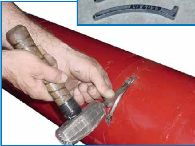
Installing Retaining Clips To Lock Casings
