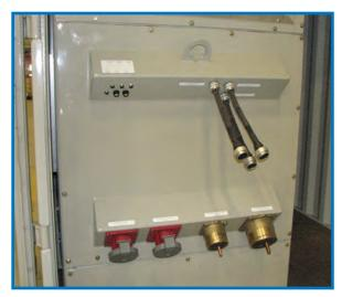
A bulkhead panel provides the connections for the electrical and communications.
