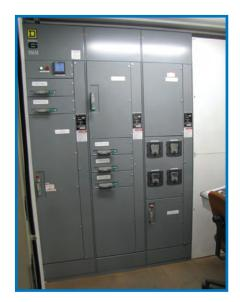
MCC (Motor Control Center) modules support and house control units, a common bus bar for power to the control units, and a network of raceways to accommodate load and control wires.
