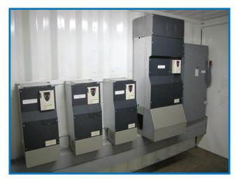
The variable frequency drives (VFDs) efficiently control the electric motors for the main MTBM drive, slurry feed, slurry booster, and slurry return systems.
