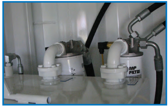
Hydraulic Filtration for Hydraulic Return & Hydraulic High Flow Return Circuits
