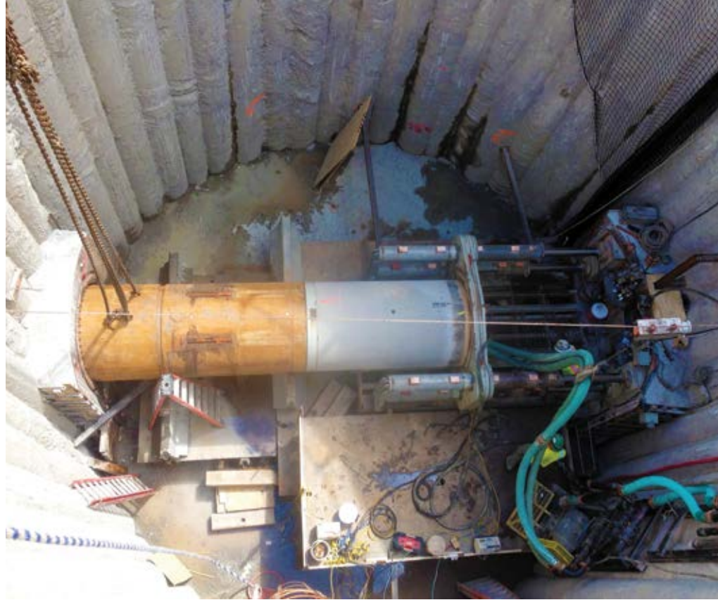
First MTBM launch August 15 2014 from a 45 foot deep secant pile shaft using an Akkerman with an MT860K jacking frame
