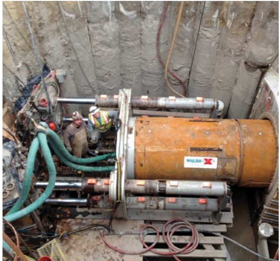
First MTBM launch August 15 2014 from a 45 foot deep secant pile shaft using an Akkerman with an MT860K jacking frame
