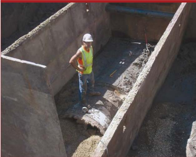
a residential area and the drive had to advance from west to east, under Highway 51. The 12x20-ft jacking pit was constructed at 20-ft deep in late August, near the shoulder of Highway 51. The drive commenced in a small stream on the east side. Crew members oper-
