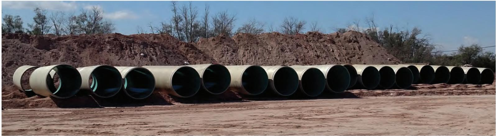
**THOMPSON PIPE GROUP IS SUPPLYING THE FLOWTITE FIBERGLASS PIPE FOR THE PROJECT.**
