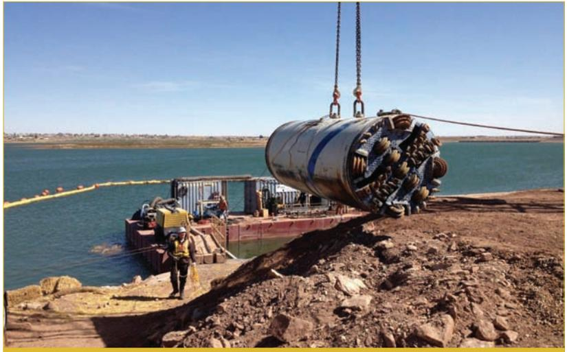
MT460 jacking frame, control container and bentonite pump with a Derrick Flo Line Primer slurry separation plant for microtunneling operations. The MTBM was outfitted with a bulkhead to seal off the sensitive internal components of the MTBM from water damage when retrieved from the reservoir. The MTBM cutterhead was equipped with disc cutters, drag teeth, and picks to meet the 15,000-psi rock cutter baseline.
