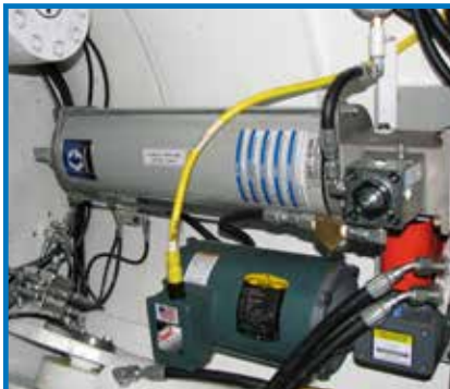
Bearing Seal Grease System
