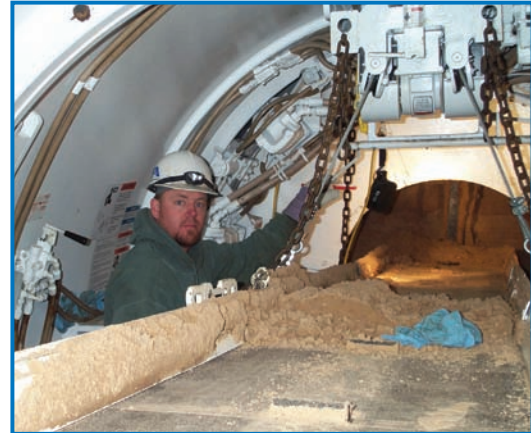
The operator station is located along the inside of the TBM wall beside the conveyor. The operator can control the TBM steering and monitor or adjust the spoil removal as necessary.
