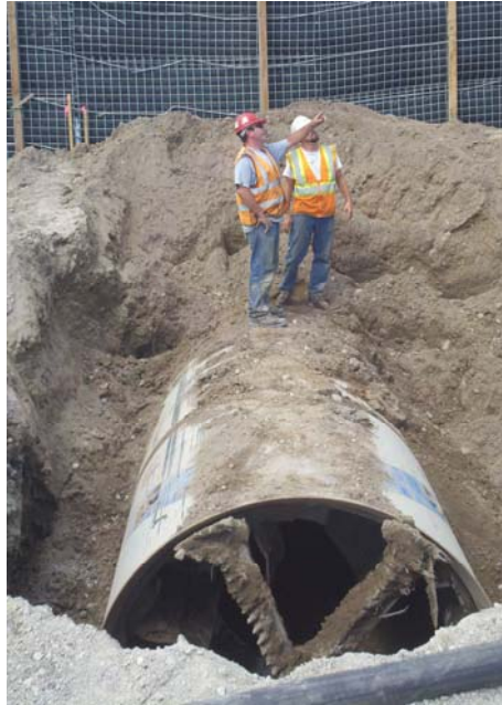
Figure 5. This TBM has emerged with little depth of cover.
