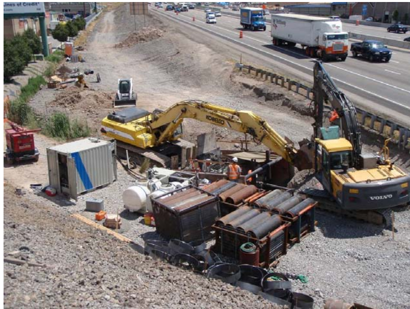
Figure 3. GBM construction work along I-15 CORE project with moving traffic.
