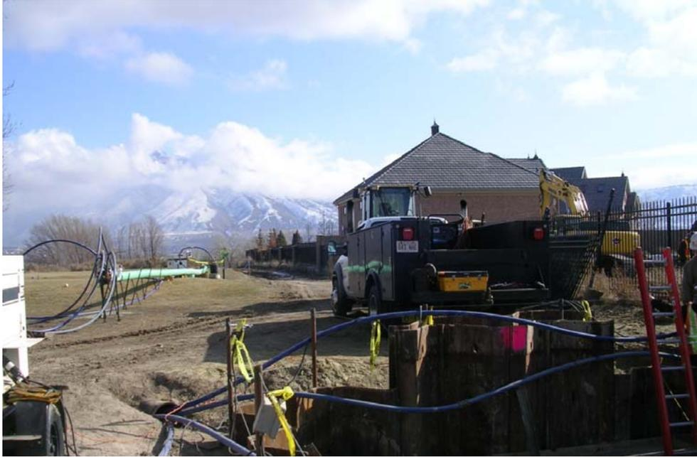
Figure 6. Dewatering along the first 480-ft alignment.
