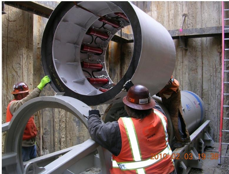
Figure 8. A jacking can is being installed between the TBM and the 5000 Series Pump Unit.
