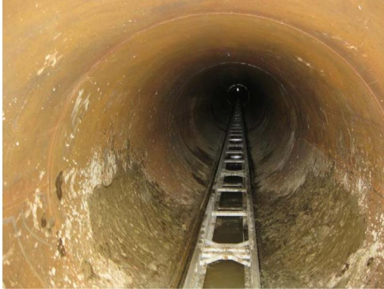
Figure 9. The completed 787-ft tunnel.
