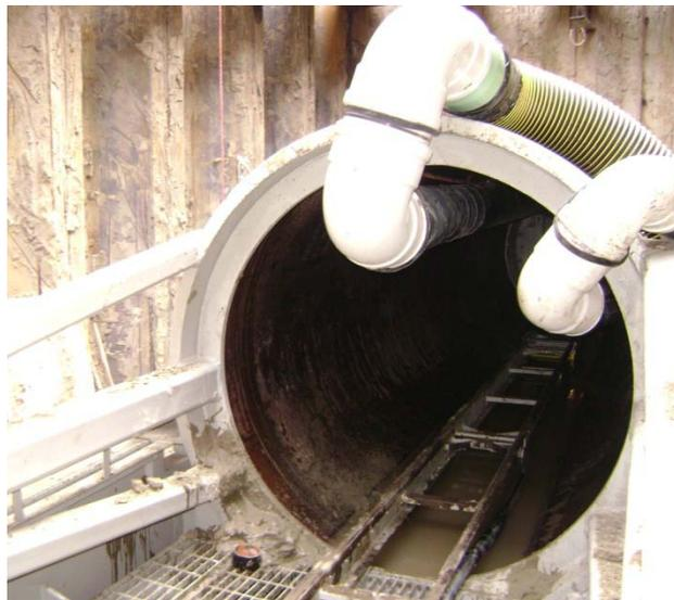
Figure 3. Tunnel ventilation duct work.
