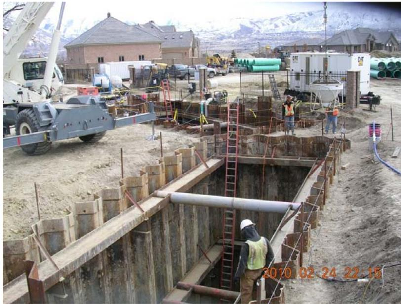
Figure 5. Construction of the second portion of the "L" shaped shaft.
