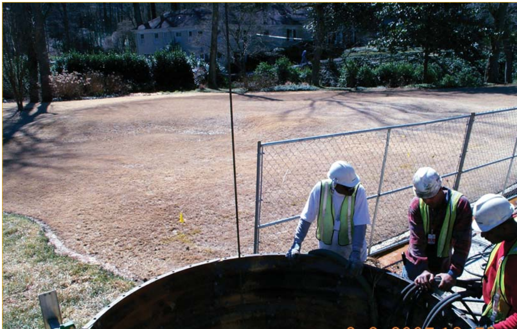
Minimized surface disruption was a huge factor on this job, since the picturesque five-acre property features a putting green on a secluded wooded lot with a creek.
