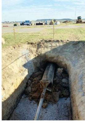
uger boring contractors have a host of convenient tooling choices for tackling the expected and even unforeseen ground conditions for common diameter steel casing installations.
