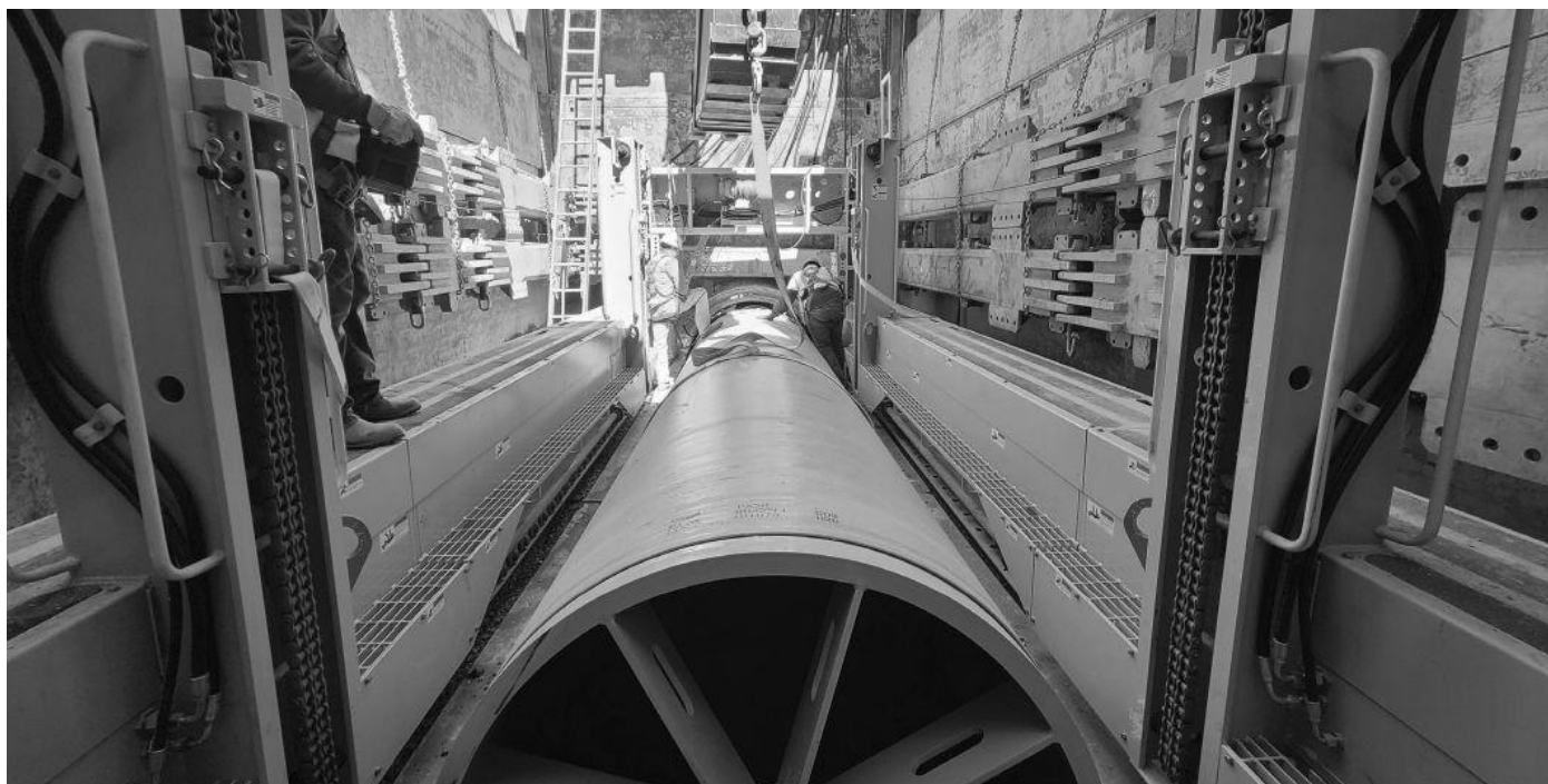
Figure 1: Hobas sliplining project in New Mexico by RMCI - A NOX Group Company
