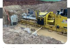
ing with wet weather and groundwater coming in from the Tennessee River. The auger boring machine was operated at idle for Akkerman GBM installation.
