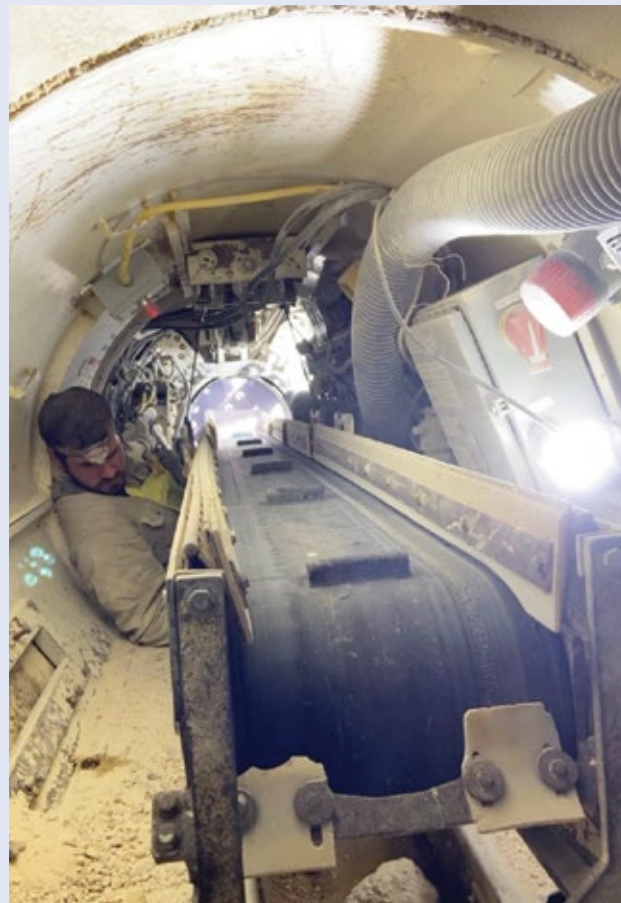
Key benefit of the Akkerman TBM is ability to access the face for obstruction removal
