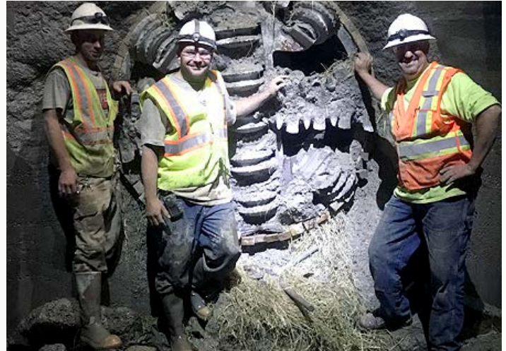
SEI's SL60 MTBM cutterhead emerges after completing a 765-ft. curved microtunneling for the NEORS. Pictured from left to right are SEI crew members Justin Okruhlica, Glen Riley and Jim Strane.
