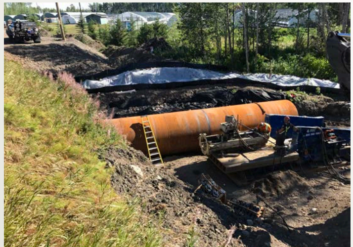
TTC was subcontracted to install a 2440mm, 45m main culvert and 1200mm overflow culvert under Highway 16 in British Columbia.
