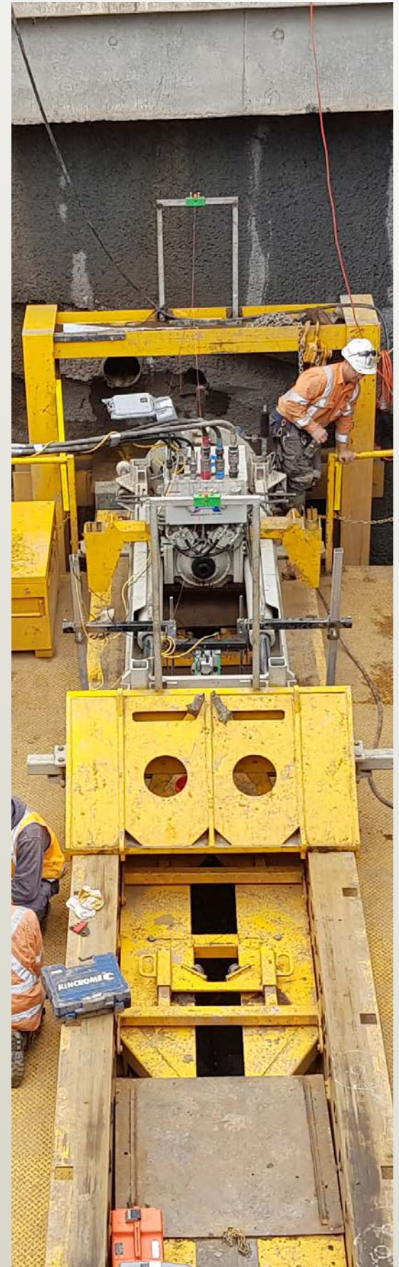
Step three in TS's process launched the 350mm diameter canopy tubes with lead integral cutter head and enclosed augers along each pilot tube bore path.
