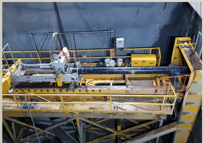
The contractor's GBM system and adjustable support and tension frame is used to install successive installations of 350mm steel casing canopy tubes.
