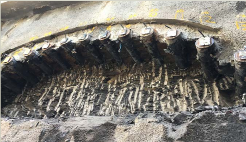
A completed pipe canopy before the installation of the of the support structure to be inserted below.
