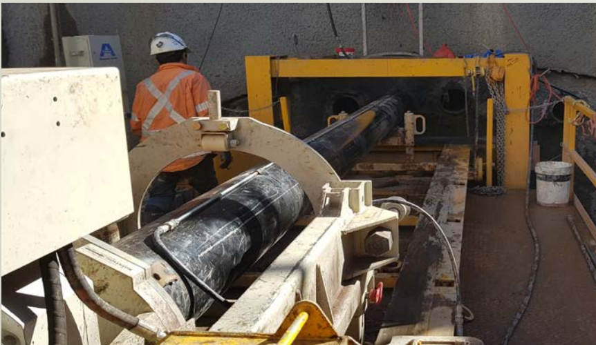
Step three in TS's process launched the 350mm diameter canopy tubes with lead integral cutter head and enclosed augers along each pilot tube bore path.
