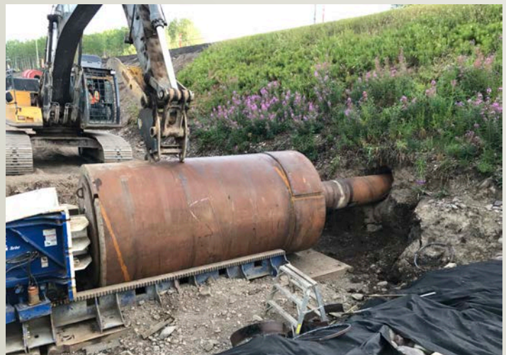
Pilot tubes initiated the 2440mm, 45m main culvert installation followed by a 760 to 2440mm adapter.
