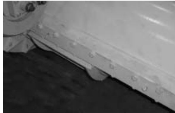
#1 Screw Conveyor Gate
