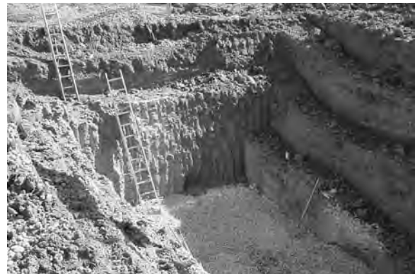
Auger Boring Shaft
