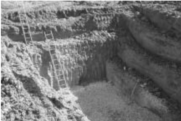
Auger Boring Shaft
