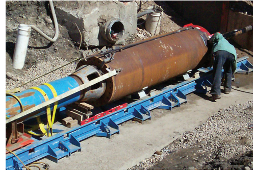
Figure 13. The first guided pipe ramming project in 2006. Photo credit Claude H. Nix Construction.
