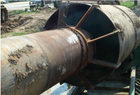
Figure 9. Upsizing to the final diameter steel casing with a two-stage WORH.
