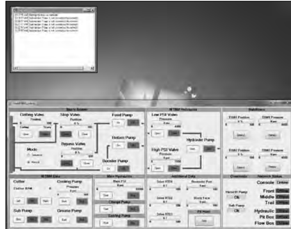
Log Message and MTBM Control Screens
