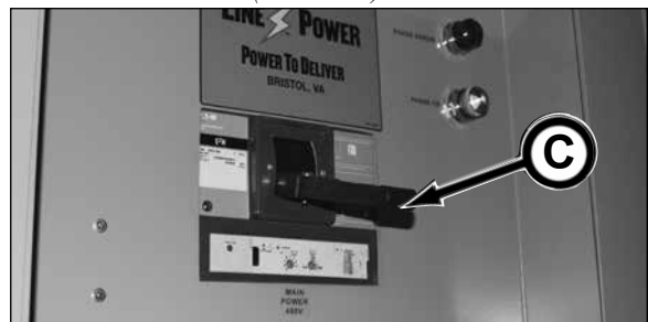
Power Container (FA22062F) Main Power Switch
