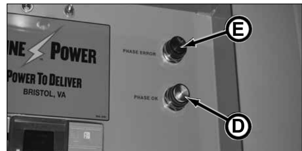
Main Drive Power Container (SN FA22062F)
