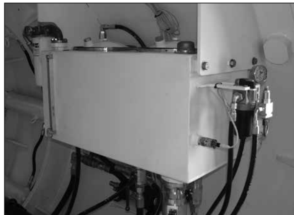
Remote Hydraulic Power Pack (FA21965F)
