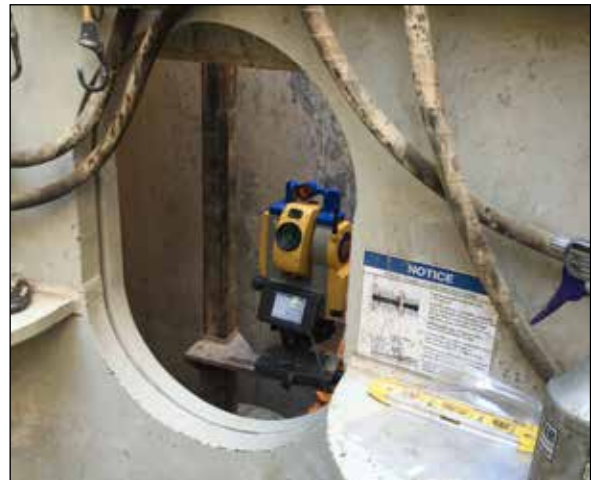
Shaft Station In Launch Shaft
