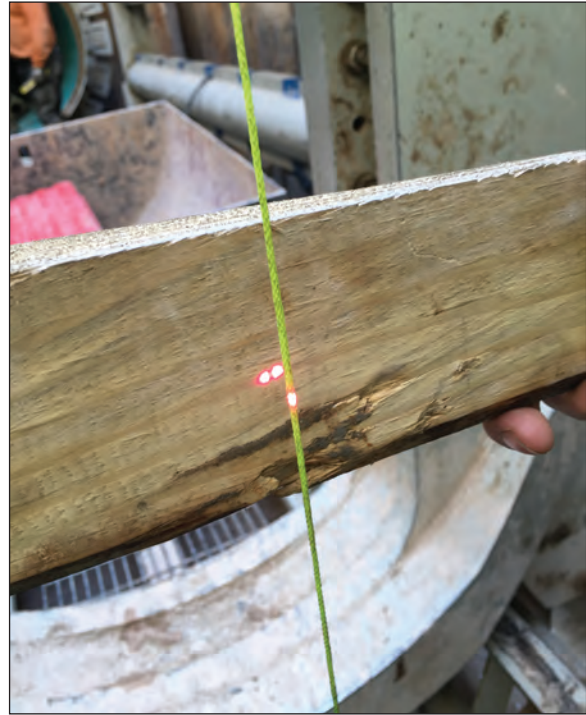
String Line In Back of Launch Shaft
