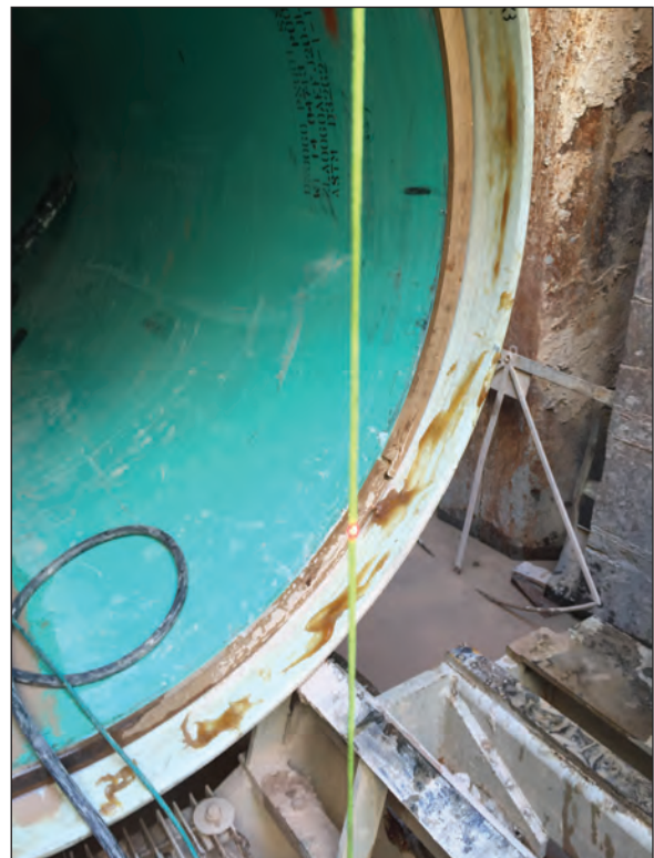
String Line In Front of Launch Shaft
