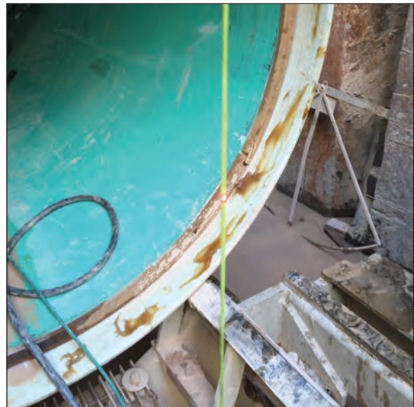
String Line In Front of Launch Shaft
