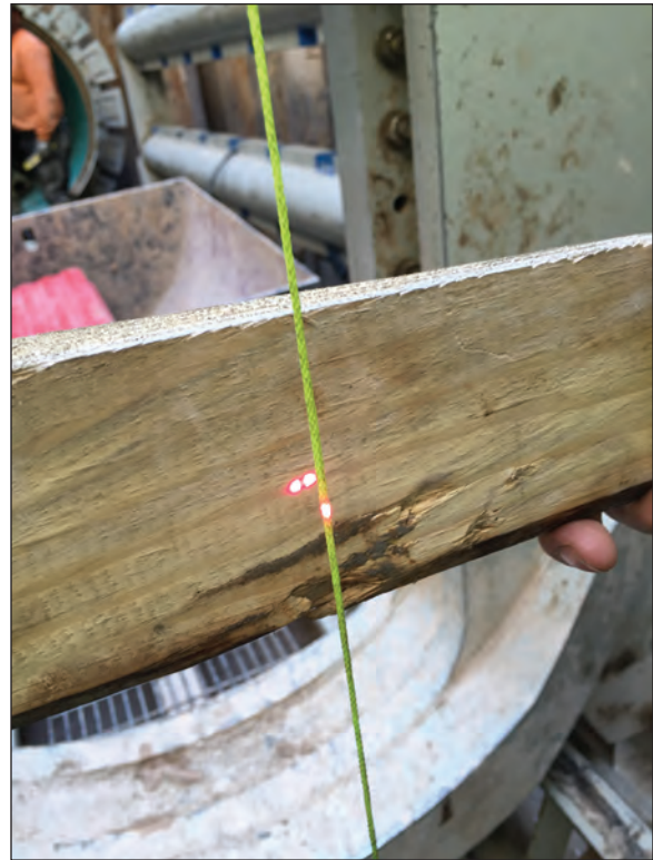
String Line In Back of Launch Shaft
