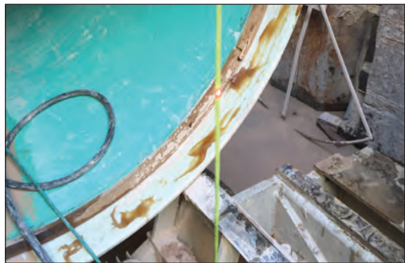
String Line In Front of Launch Shaft
