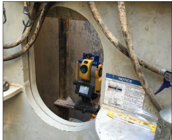
Shaft Station In Launch Shaft
