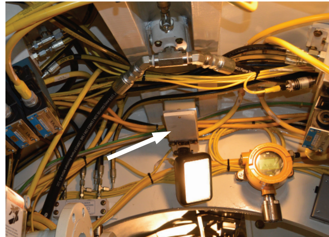
Figure 17. Front MTBM inclinometer; one of three.
