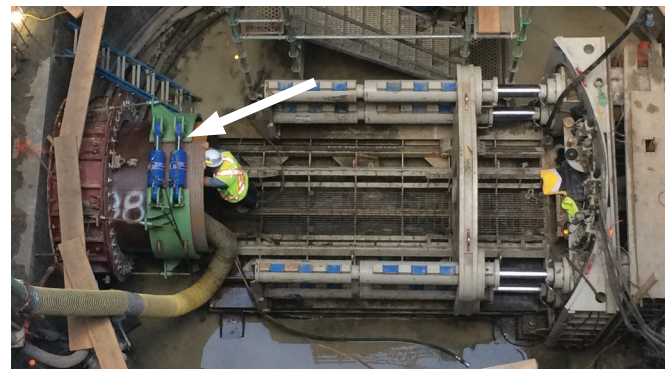
Figure 15. A pipe clamp is used when microtunneling within a body of water to hold the previous pipe segment in place and contend with buoyant forces.
