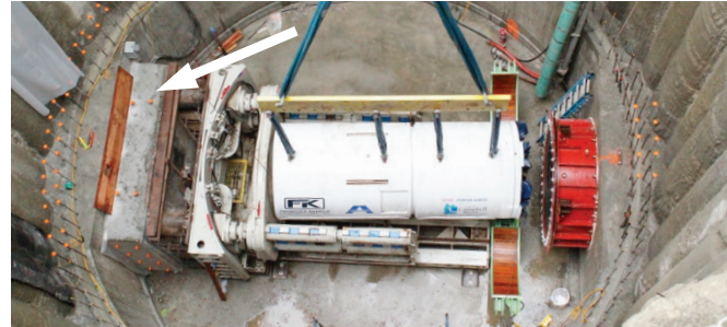
Figure 9. Concrete reaction wall is poured at the rear of the jacking shaft to disperse jacking loads.
