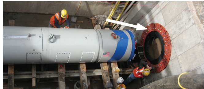
Figure 10. The MTBM is typically launched through a shaft seal to prevent subsidence from entering the launch shaft.
