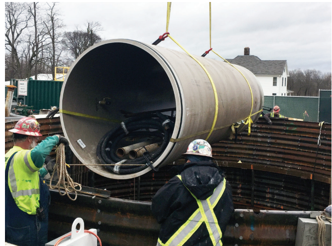
Figure 13. As pipe segments are lowered into the launch shaft, microtunneling utility lines are lowered inside the pipe and are connected to the existing lines.
