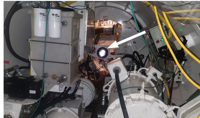
Figure 18. The MTBM active target is mounted in the back center of the MTBM.
