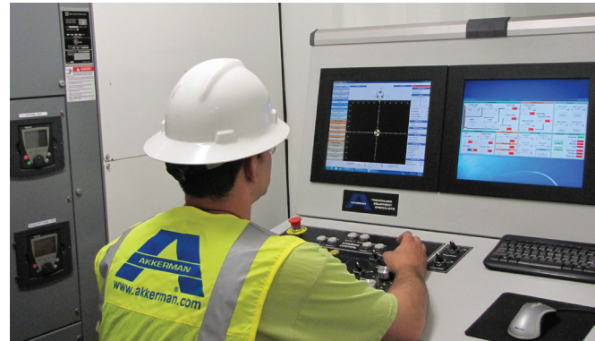
Figure 1. Microtunneling systems are remotely controlled from a control console inside the control container on the surface.
