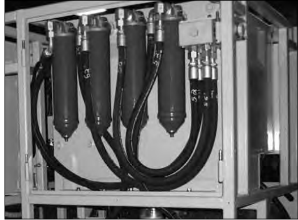
Boring Head Hydraulic Reservoir
