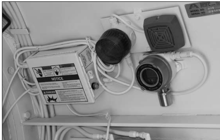
Akkerman Methane Gas Detection System
