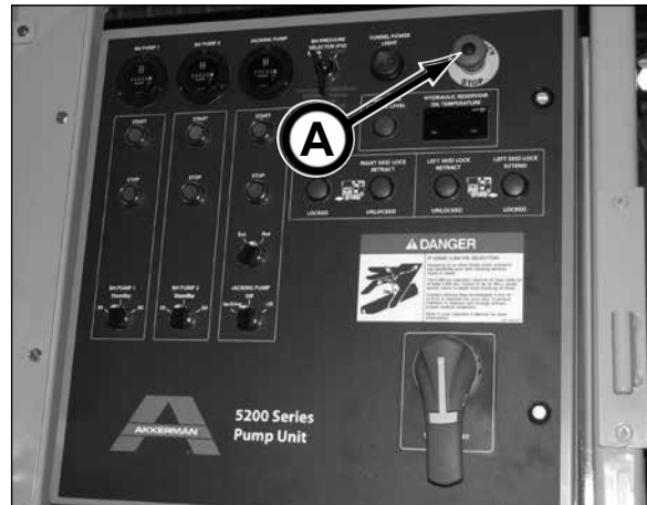
E-Stop on 5200 Series Pump Unit
