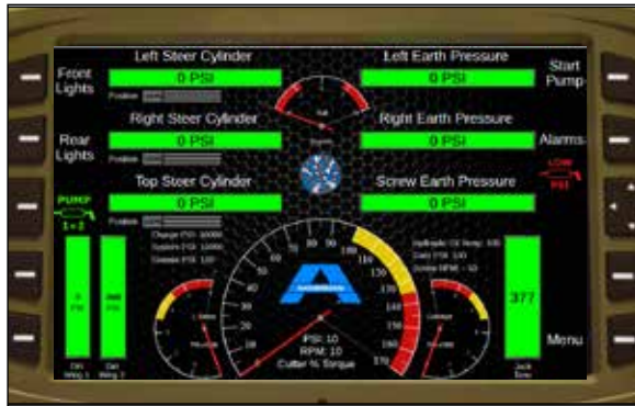
Main Control Screen
