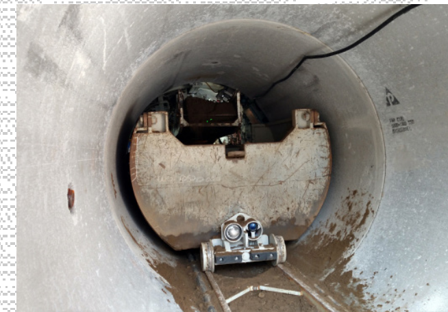
Figure 11. Dirt bucket and haul unit on a track.
