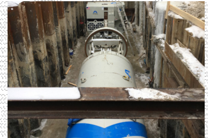
Figure 8. The Tunnel Boring System is an all-in-one pipe jacking solution.
